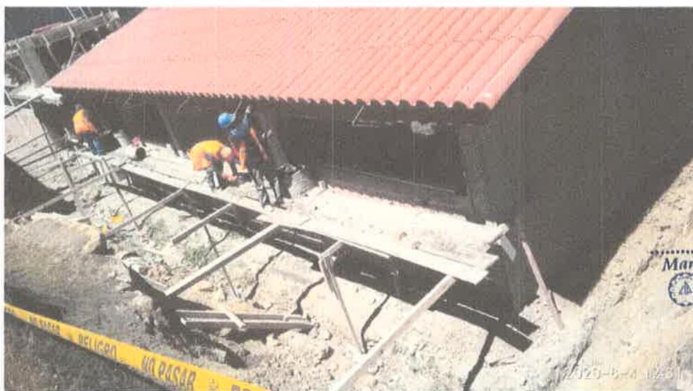
**FOTO 4: TARRAJEOS EXTERIORES EJE 3 TRAMO (A-D) MODULO III**
