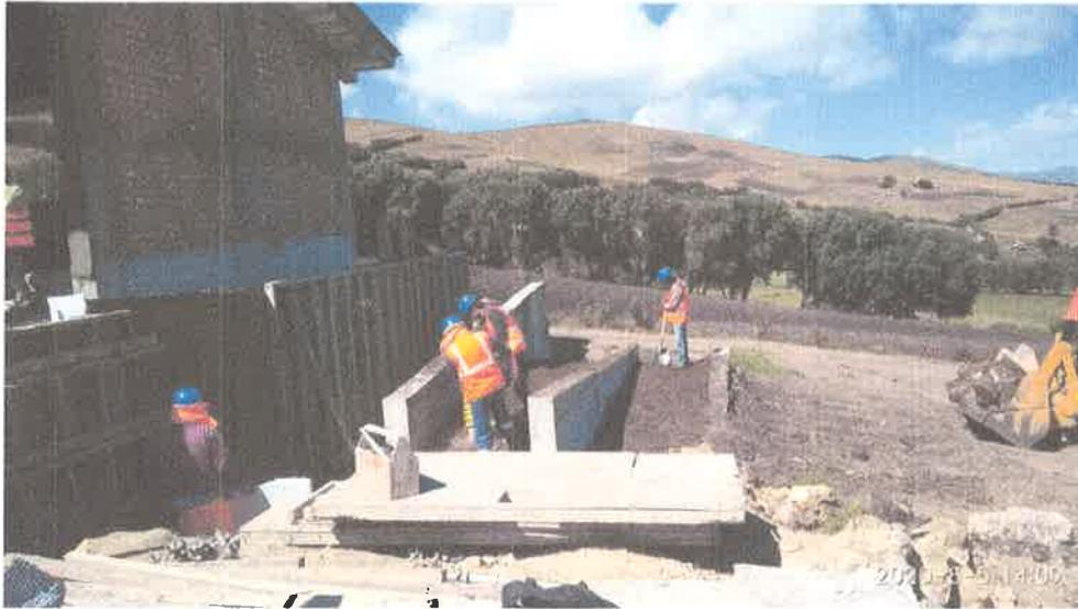
**FOTO 5: RELLENO Y COMPACTADO CON MATERIAL PROPIO EN RAMPA**
